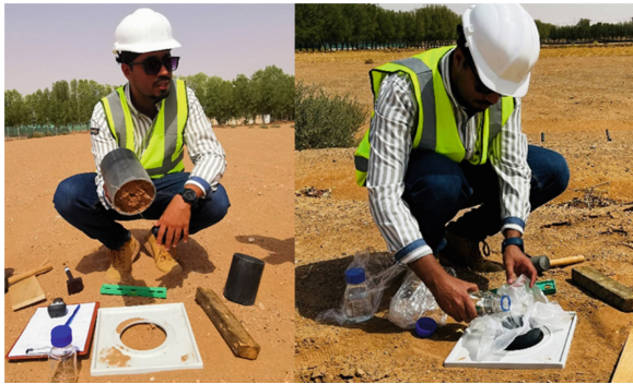
Fig. 1. Onsite soil infiltration test.
